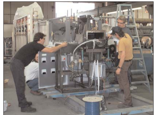
Harper employees test and assemble electrical system to furnace.
